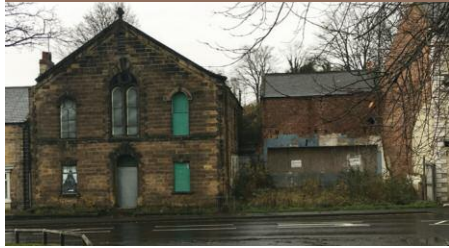
Clearing the dilapidated site to make way for future sustainable development.
