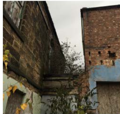
4 / View between Chapel and School house
