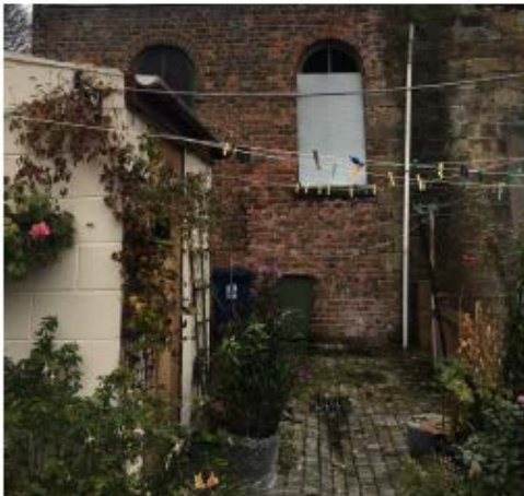
3 / View of Chapel from rear
